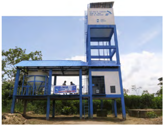
The whole system is activated by solar energy
