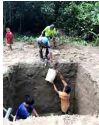
Nuevo Progreso: the digging of the artisanal well, filling the trenches and transporting cement from the river to the village.
