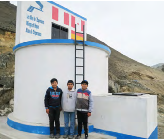
The Rio Seco reservoir topped by the chlorination caseta
