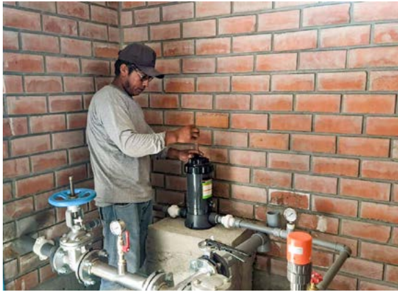
Venturosa: Maestro Llutari installing the water chlorination system
