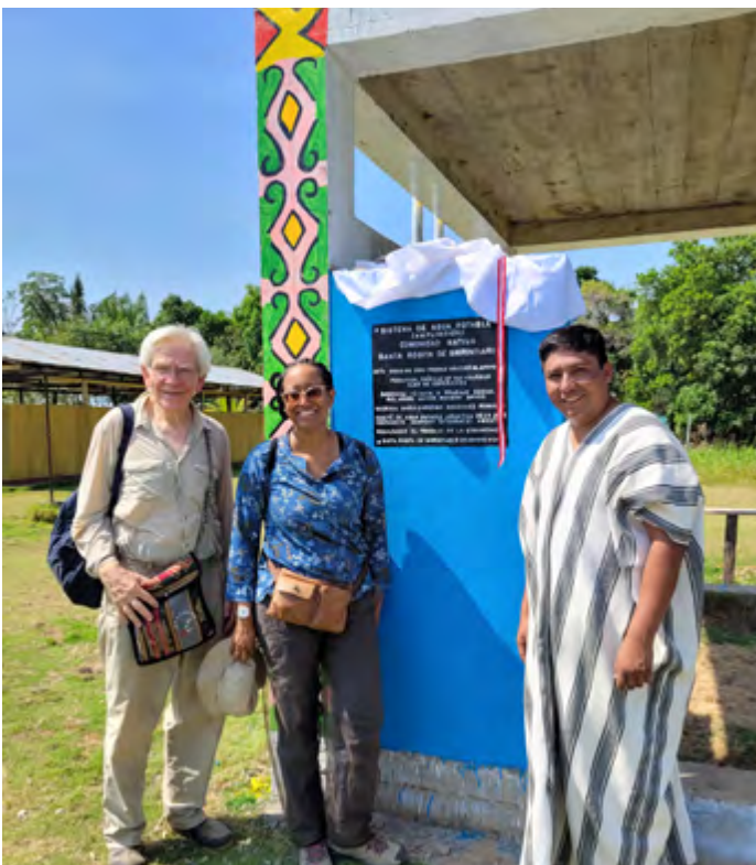
Santa Rosita de Shirintiari: André Franche, María-Christina and the engineer Ángel Huaman in front of the beautifully decorated reservoir, now a tourist attraction!
