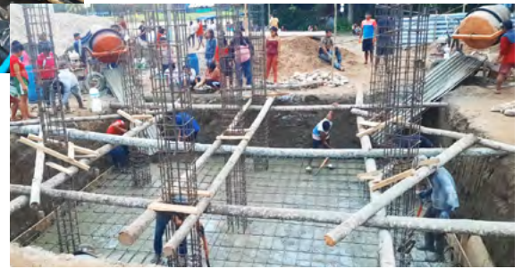
Building the reservoir base
