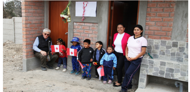
Our Peruvian team returned to Nueva Esperanza to install a water inlet at the nursery school and build an eco-friendly toilet for the children.
