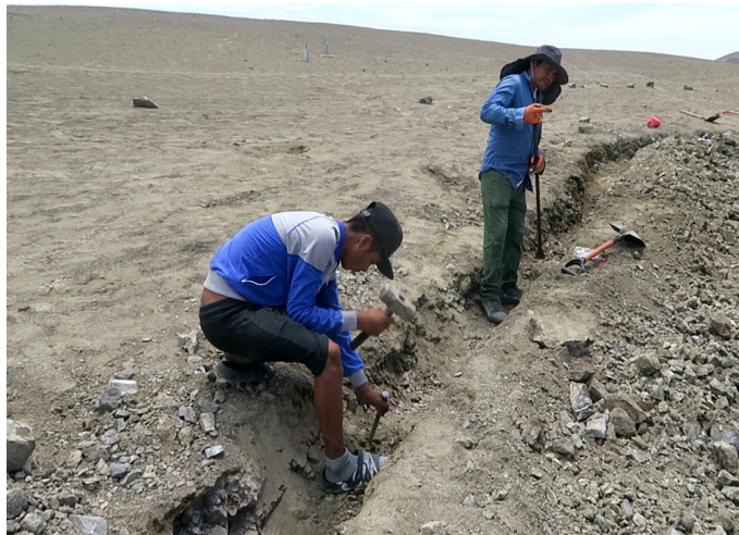
Digging a trench in rocky soil
