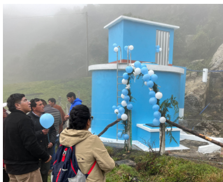
The cistern in Alto Verde
